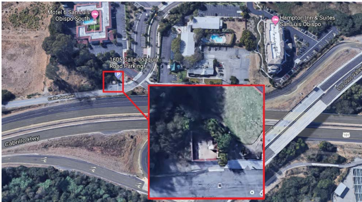
FIGURE 19 CALLE JOAQUIN PUMP STATION PROXIMITY TO LOCAL HOTELS
