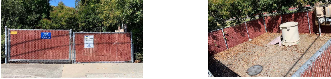
FIGURE 17 CALLE JOAQUIN PUMP STATION
