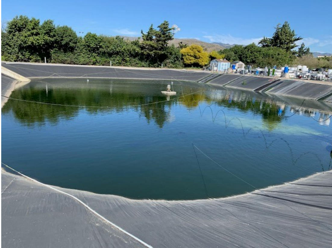
FIGURE 14 OVERVIEW OF LAGOON SYSTEM AND HIGHLIGHT OF NON-BUOYANT OXYGEN INFUSION TECHNOLOGY
