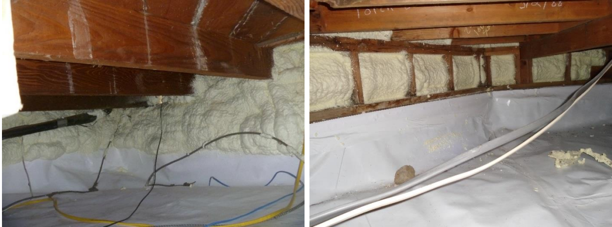
FIGURE 3 – VAPOR BARRIER AND INSULATION AFTER MEASURE IMPLEMENTATION
