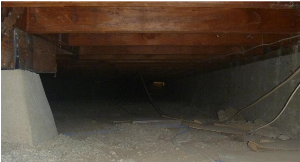
FIGURE 1 – UNCONDITIONED, VENTED CRAWL SPACE EXAMPLE
